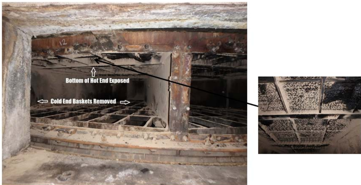
Figure 3: Hot End Air Heater Baskets.
